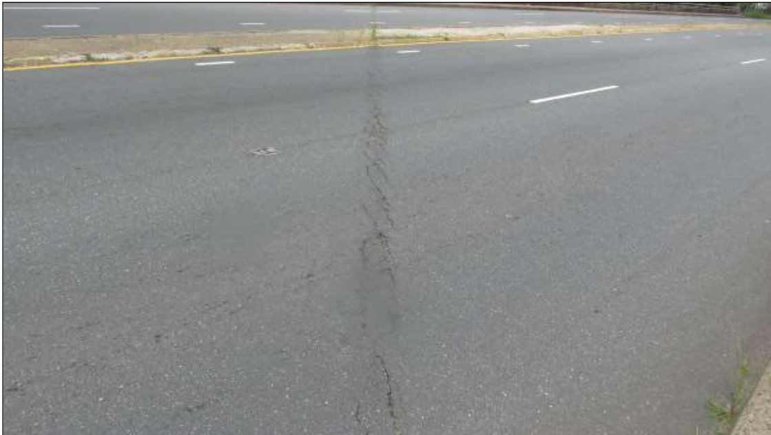
ASPHALT WEARING SURFACE CRACKING OVER THE INT. BENT JOINTS.
