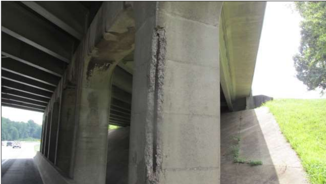
COLUMN 7 AT BENT 3 HAS A CORNER SPALL ON THE SOUTH FACE FOR 7' HIGH X 5" WIDE WITH REBAR EXPOSED.
