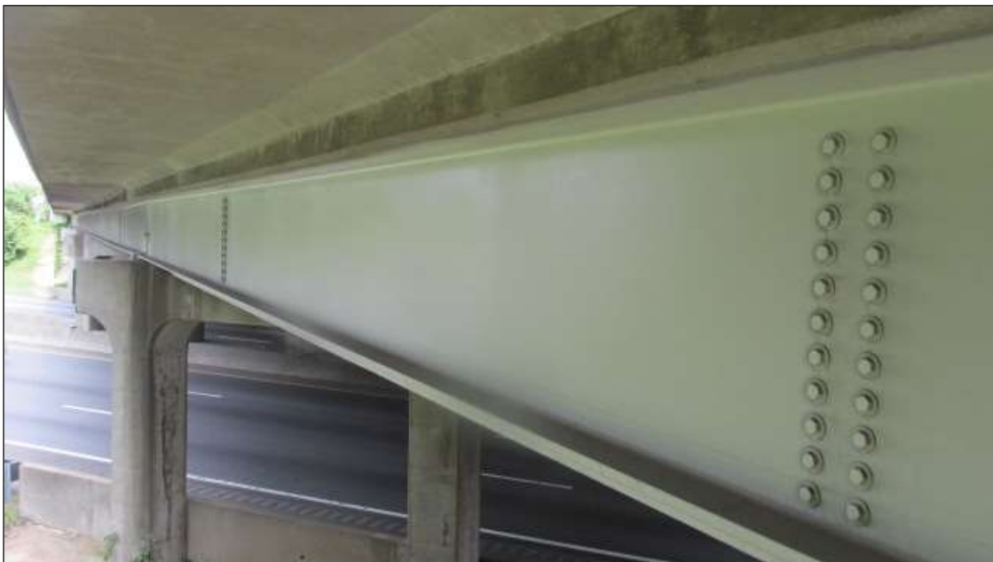
STEEL PAINTED IN RECENT PAST.
