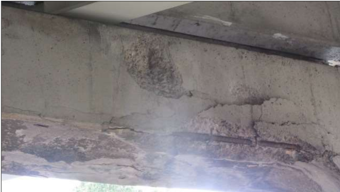
THERE IS A 14" WIDE X 12" HIGH CONCRETE SPALL WITH RBAR EXDPOSED UNDER BAY 13 BENT 1 WEST FACE. ALSO THERE IS A 7' WIDE SPALL ALONG THE BOTTOM CORNER
