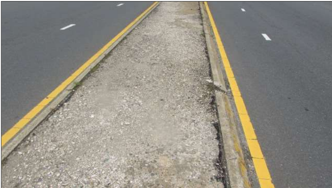
THE CONCRETE MEDIAN. IS DETERIORATED AND CRUMBLING.
