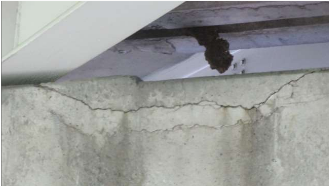
H/L TO 1/8" CRCK ALONG THE TOP CORNER OF BENT 3 CAP EAST FACE ADJ. GIRDER 9 FOR 3' ALONG THE TOP CORNER.
