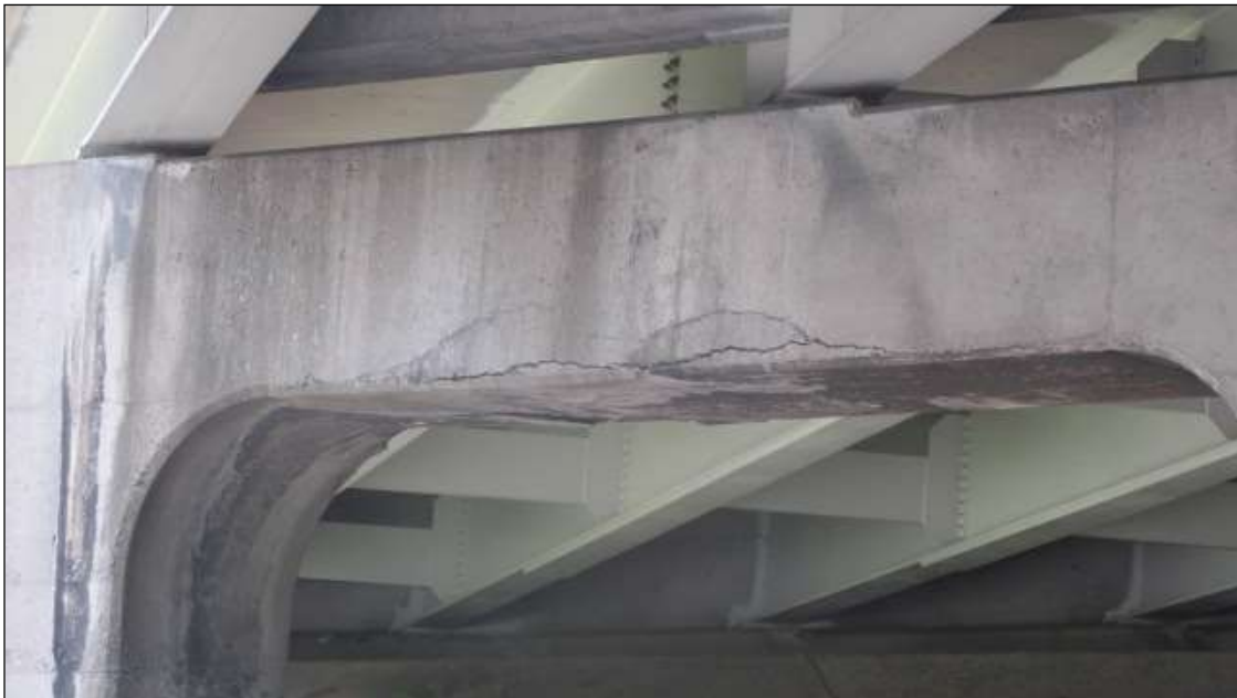
SPALL ALONG THE BOTTOM CORNER OF BENT 1 EAST FACE UNDER BAY 1 FOR 5'
