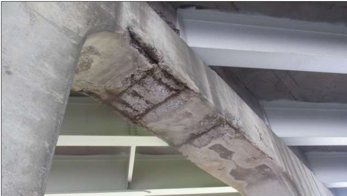
THE BOTTOM OF THE BENT 3 CAP BETWEEN COLUMNS 5 AND 6 HAS SPALLED 3' W X 3' L X 2 1/2" DEEP WITH RBAR EXPOSED. A PRIORITY MAINT. ISSUED.
