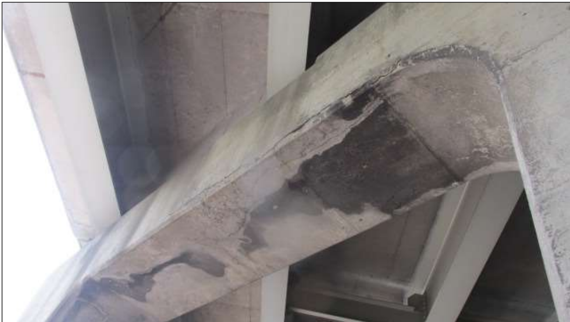
H/L TO 1/8" CRACKING ALONG THE BOTTOM CORNER OF BENT 2 IN BAY 1 FOR 4' ON THE WEST FACE.
